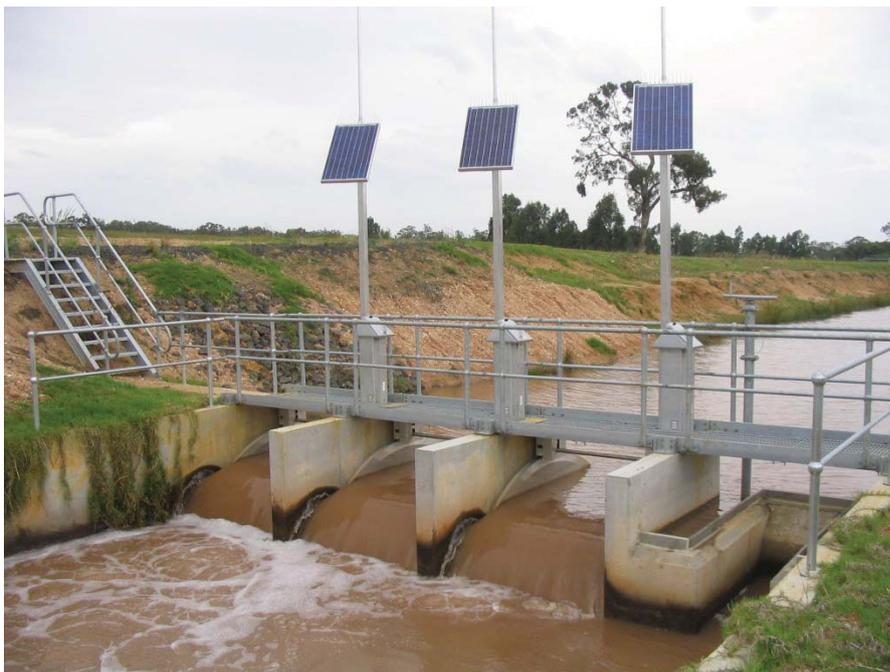
Figure 13: Picture of gates at 877A powered by solar panels
