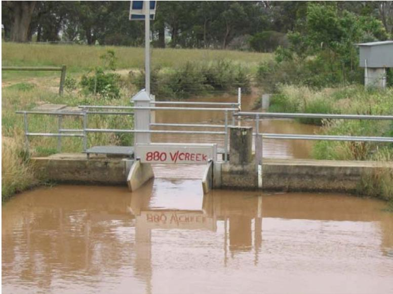
Figure 10: Picture of the offtake at gate 880
