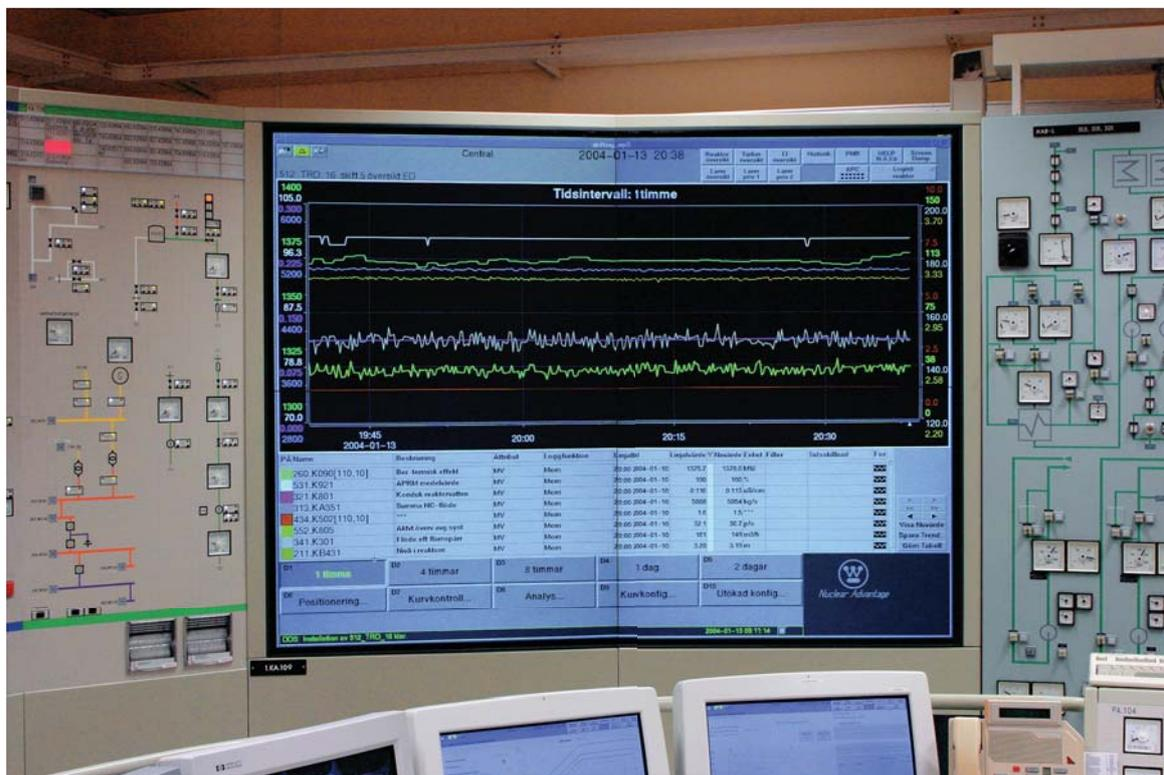
Figure 4. The large screen display in the nuclear control room, fitted in between the security panel (left) and the turbine wall panel (right).
