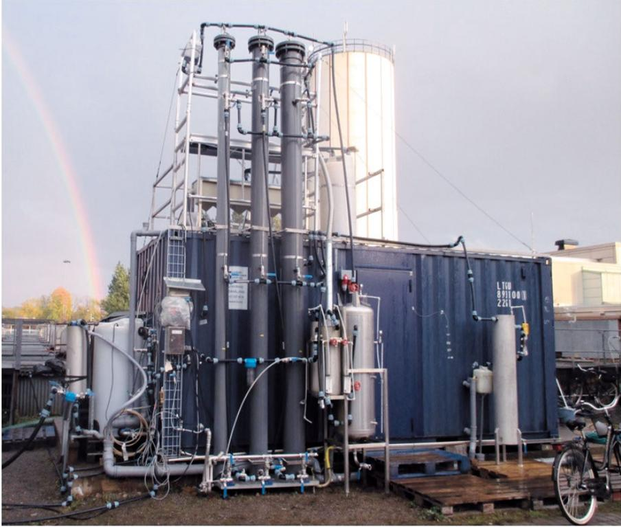
*Figure 6.* The pilot plant with technology for additional treatment of STP effluent developed by Berndt Björleinius at the Royal Institute of Technology, Stockholm. (Photo by Berndt Björleinius).
