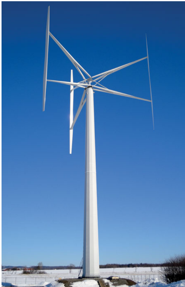
Figure 2.2. The three bladed 200 kW vertical axis wind turbine in Falkenberg, Sweden.
