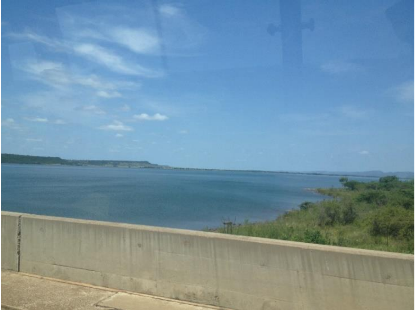
Fig 14. Piquenos Libombos Dam visited 19 th of February 2015, photo taken by the author.
