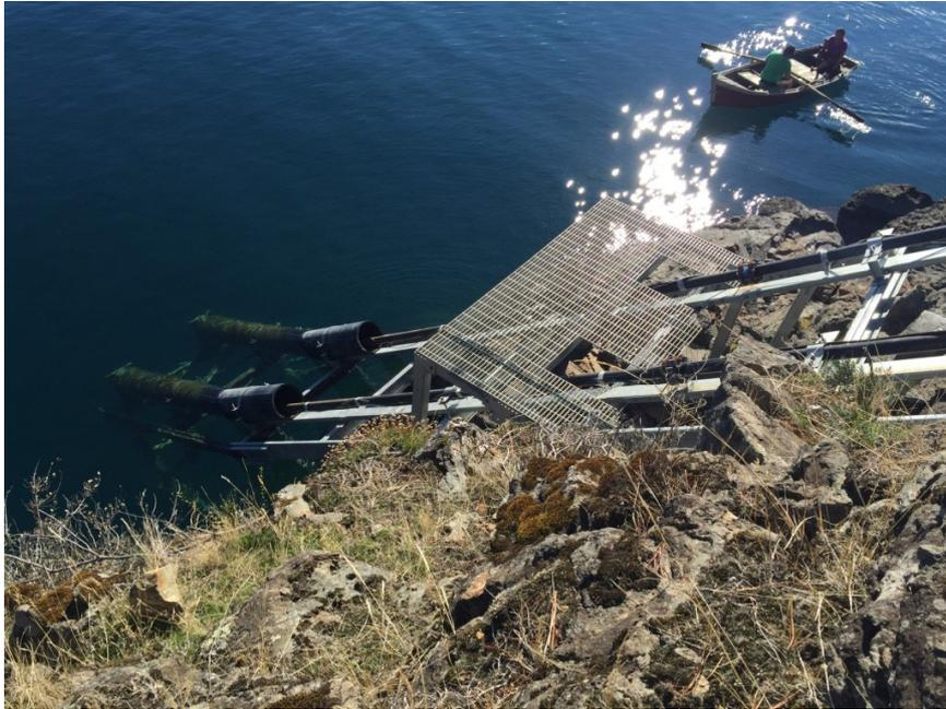
**Fig. 2.** The water pumps hanging in the air above the water surface, making it impossible for the water to enter the irrigation system. Photo: Martine Greek.
