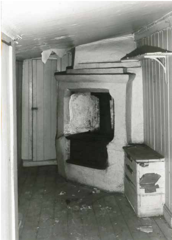
Figure 7.9 Hunnebergsgatan 7, a small kitchen preserved on the second floor, representing a later addition in the built-in open gallery. Documentation from the 1970s, Archive of Östergötland's museum.
