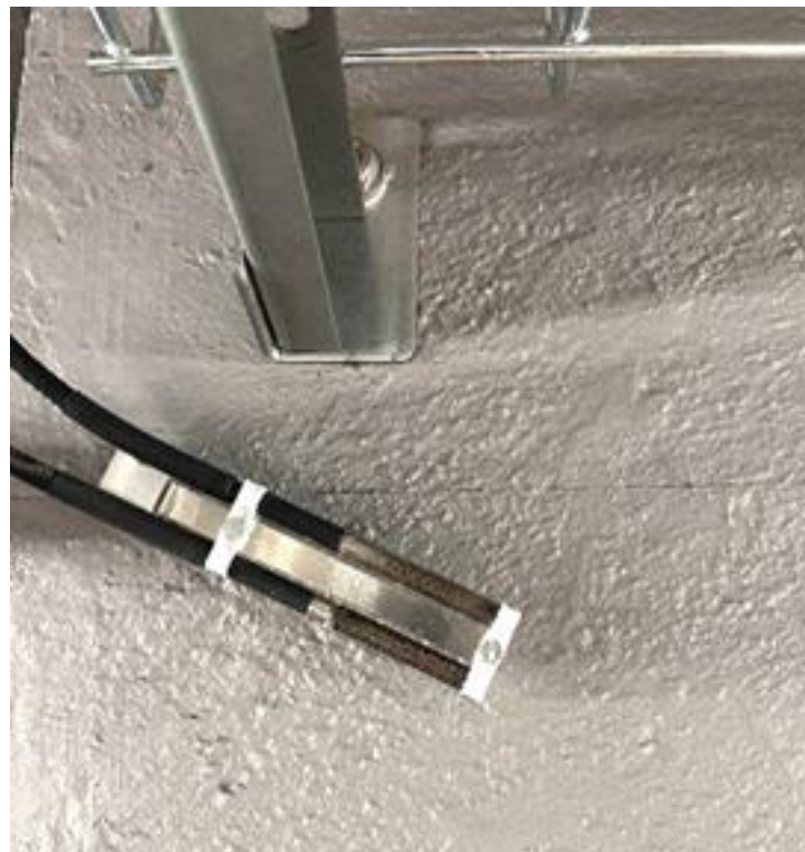
Figure 5. The pair of uFC placed in a simple holder made of thin plastic components on a thin Al base plate. Here the pair is mounted on the wall of the NESSA inner bunker, in a position known as the FC-IB. See Section 5 for further details on the measurements in this position.
