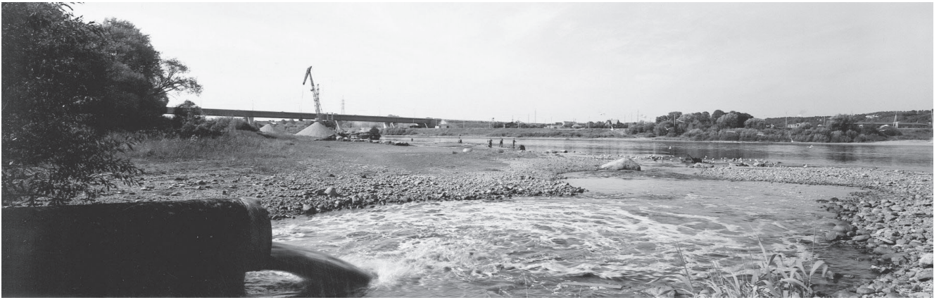
Figure 17.10. From this pipe 70% of the wastewater from the city of Kaunas, Lithuania, in the early 1990s, came out in the river untreated. The situation was similar in most cities in central and eastern Europe. Kaunas, Lithuania’s second largest city, has more than 400.000 inhabitants. The wastewater treatment plant is now expanded, with financing from among others the Swedish International Development and cooperation Agency. (Photo: Victor Brott, courtesy of Sida.)
