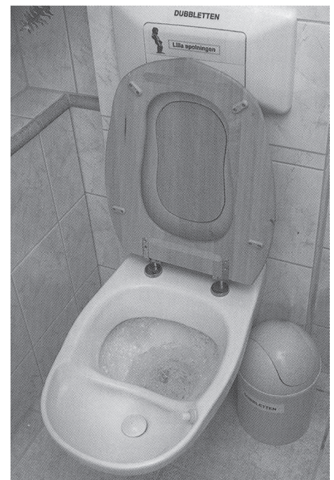
Figure 17.34. A urine separating toilet. In this kind of toilet urine is collected separately, and used after storage as fertiliser in agriculture. The urine contains most of the nitrogen and is sterile. (Photo: Per G. Berg.)
