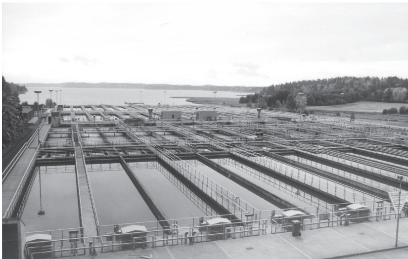
Figure 17.16. Himmerfjärden wastewater treatment plant. This plant located in the south-western part of Stockholm region receives wastewater from nearly 250,000 people. It is today highly automated. (Photo: Józef Trela.)
