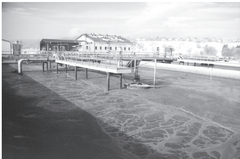
Figure 17.28. Nowy Targ wastewater treatment plant. The plant was constructed with Polish-Swedish co-operation (Swedish International Development Cooperation Agency, Sida) in 1995 and has been used by researchers from both countries studying and developing wastewater treatment technology. (Photo: Jozef Trela.)
