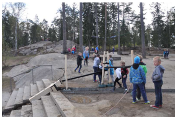
Figure 4: The tube installed at the water location.
